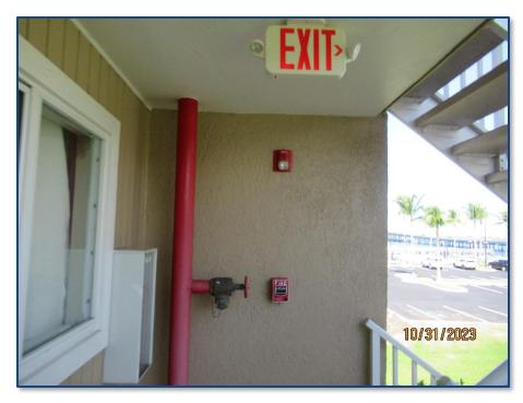
Photograph No. 29: Fire protection plumbing system, emergency exit sign, and fire alarm pull station.
