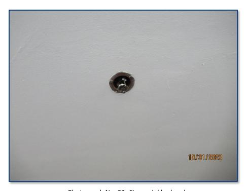
Photograph No. 32: Fire sprinkler head.
