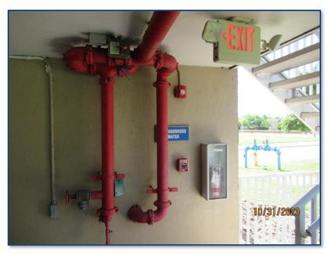
Photograph No. 41: Fire protection plumbing system.
