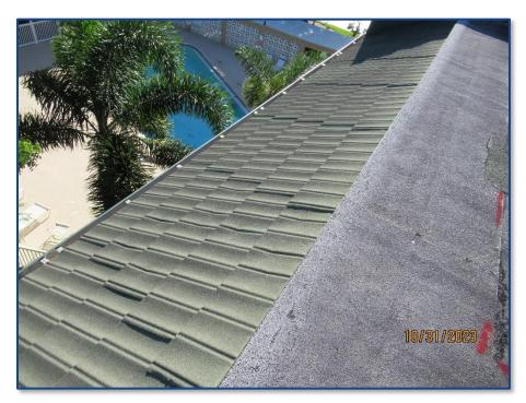
Photograph No. 16: Partial view of the mansard metal roof panels.
